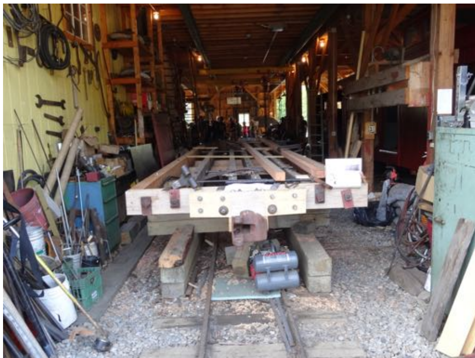
NGPF funded boxcar restoration underway in Alna, Maine
